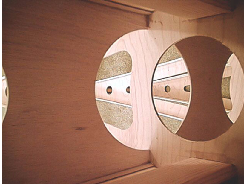
Figure 5-47 Plywood shear webs join the leading edge skin and upper and lower spar caps. Lightening holes are cut in the shear webs. Note the distance between the rear of the spar cap and the shear web. This is because this is the lower section, and the stub-mast will fit just inside the circular opening in the rib. After the load test, the spar cap was extended back to the sheer web and the sheer web reinforced with thicker plywood.
