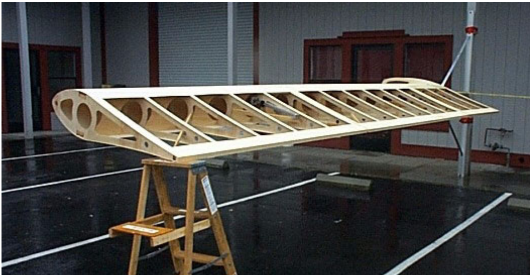
Figure 5-48 The final wing assembly setup for load testing, before covering. The ladder is only supporting the rear edge of the wing from rotating downwards (as the wing is attached to the stub-mast via bearings). The diagonal internal brace just above the ladder is the anti-drag bracing. A 72 kg load was suspended from the end of the wing, and the deflection was recorded to be approximately 15 cm. After corrections were made, the residual deflection was 5 cm.
