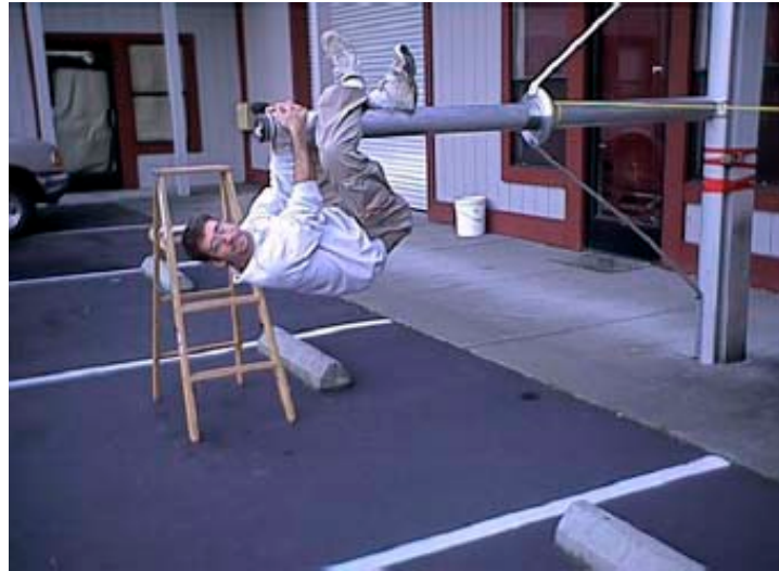
Figure 5-43 Stub mast, two spider legs, and cross beam load tested with a 72 kilogram static dummy load. The stub-mast is attached to a replacement crossbeam that is secured to a wooden column supporting the building. The two spider legs are secured to the crossbeam. Close inspection of the figure shows the two spherical roller bearings at the end of the stub-mast. No deflection occurred in the stub-mast, though the wooden column was deflected under the test load.
